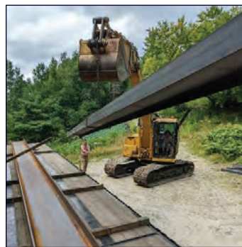
Steel being set for new bridges on Hardy Country trails.
